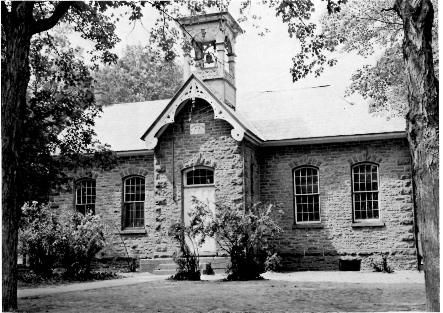
129 Maple Wood School in Oxford Mills, Oxford township. The decorative bell tower, bargeboard and beautiful setting in a grove of trees enhance the charm of this two-room schoolhouse constructed of stone obtained from a nearby farm. ( Canadian School Studios. )
